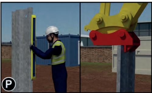
**P** The guide plates on the Drivesafe can be used to re-align the sheet as it is being driven.
