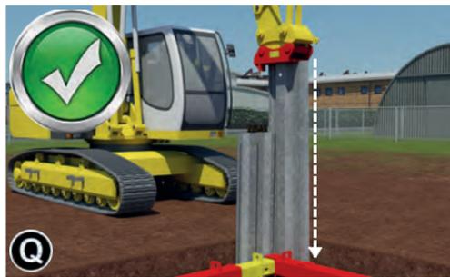
**Q** The sheet should be driven using a slow, steady push.
