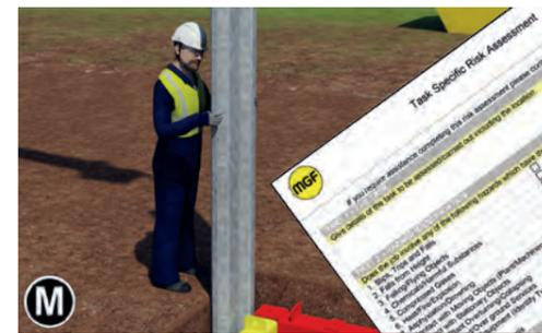
**M** Once the sheet is correctly positioned and grounded the operative may approach to assist with alignment - ensure operative follows site specific RAMS at all times during installation.
