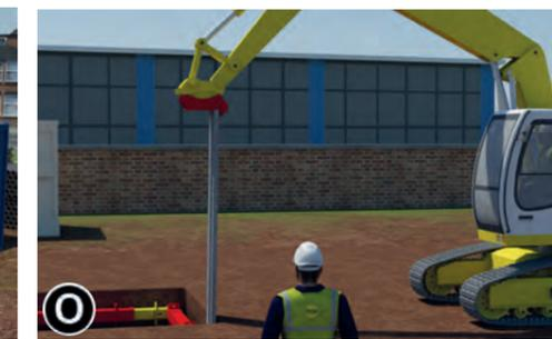
**O** The Drivesafe unit should now be used to drive the sheet to its initial level, as specified by the design.
