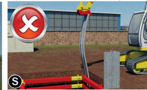
**S** If the sheet is not driving any further do not force it, as this could cause damage to the sheet and equipment.
