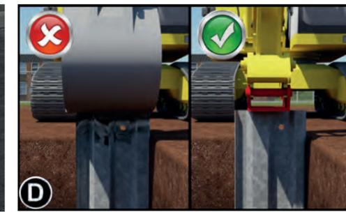
**D** Using Drivesafe reduces damage to the trench sheets and quick couplers over traditional push and dig methods, speeds up the installation process and eliminates the need for working at height.
