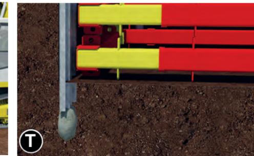
**T** Any obstructions may need removing or the excavation level may need to be reduced before driving the sheet further.
