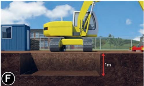
**F** Prior to attaching the Drivesafe unit the excavation is normally dug to no more than 1m in depth and the hydraulic bracing frames lowered into the trench to be used as a guide during the driving of the sheets.
