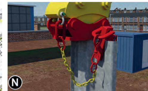
**N** Push the sheet gradually into the ground to ensure it cannot slip prior to the quick release shackle being released. Make sure the quick release shackle is out of the way of the Drivesafe so it is not damaged.
